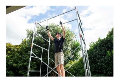
9. To do the other side, move the bottom plank up one level, and using the other plank as fall protection, place this on the top rung on the other side to install the second handrail.
