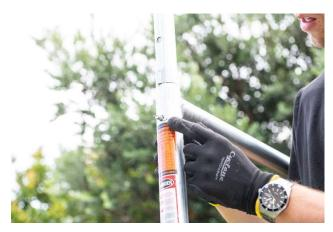
7. Lift the upright handrails into place, sliding them down on top of the joiners, fixing each one again with a bolt and retaining pin. This is the same process if you are adding another ladder frame.
