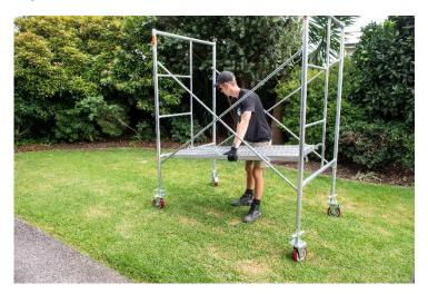
6. The plank will hold the frame square and give you a platform for lifting handrails or further ladder frames into place on top. While standing on the plank, place joiners inside each of the corners of the ladder frames and secure these with the supplied bolt and retaining pin.
