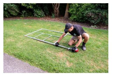
3. Find the first diagonal brace and attach both ends to the ladder frame, do the same for the second diagonal brace on the other side. Leave the other ends sitting on the ground for now. These will hold the frame up.
