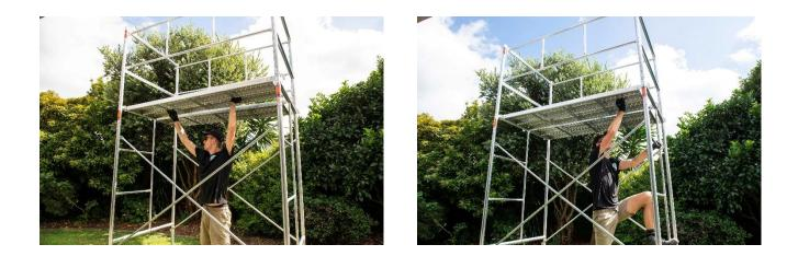
11. With your handrails fixed in place and castor brakes on, you can begin to use the scaffold tower. To dismantle, just reverse these steps. To build the double height tower, follow the same process, moving planks up and ensuring you are protected by fall protection as you go.
