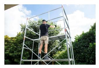
10. Finally, move the planks to the desired level. Be sure to place the trapdoor plank on the side with the ladder rungs. This will be accessed by climbing internally.
