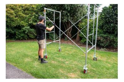
5. Once both ladder frames are secured to the diagonal braces, your scaffold will be able to stand on its own. It is a good idea now to check the tower for levelness and adjust where necessary. Place a plank onto the first level of the scaffold.
