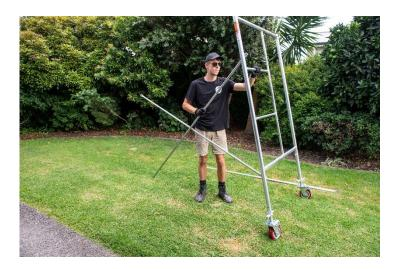
4. Find the second ladder frame and in the same fashion slide the wheels inside. Move frame and wheels to the other end of the diagonal braces sitting on the ground and attach them by picking up the ends of the diagonal brace and sliding them onto their retainers.
